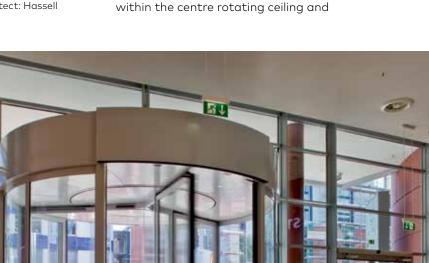
breakout door wings for alternate access
